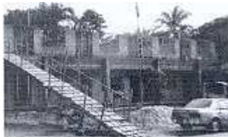
The 2nd floor of the three-story building now at decking stage
